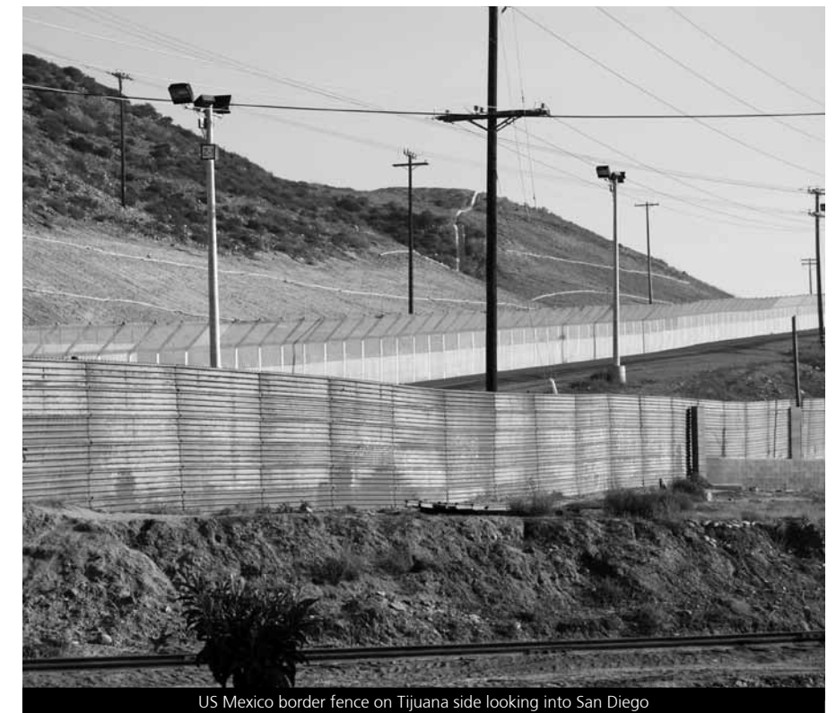
US Mexico border fence on Tijuana side looking into San Diego
